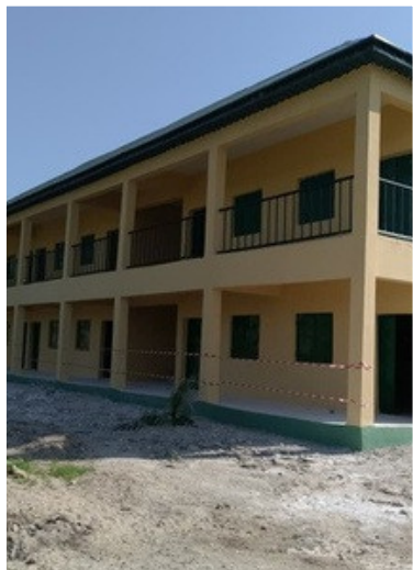
New blocks of classrooms at Government Secondary School Bukuru built by the AGILE project in Plateau State
