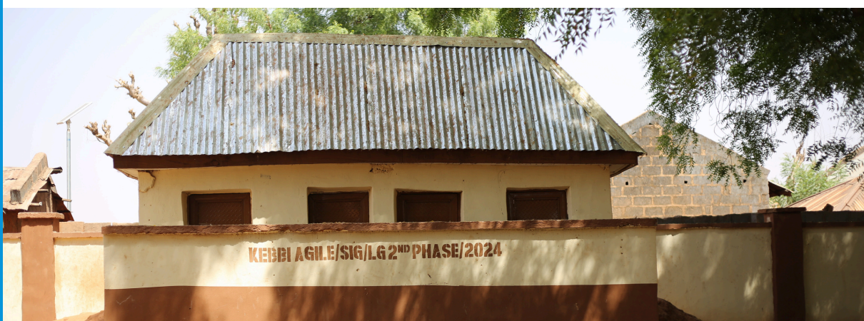
Newly constructed toilet facilities by AGILE at Government Day Secondary School Alelu, Kebbi State
