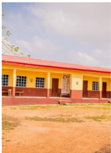
Newly renovated block of classrooms by the AGILE Project in Ekiti State.
