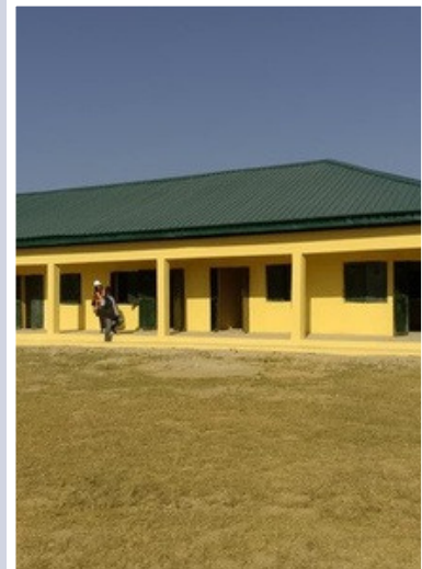
AGILE project in Plateau State finishing renovation of blocks of classrooms at Government Secondary School, Giring Abatuwa
