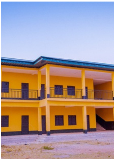
Newly constructed block of classrooms by Kaduna AGILE at Government Junior Secondary School, Kakuri Gwari
