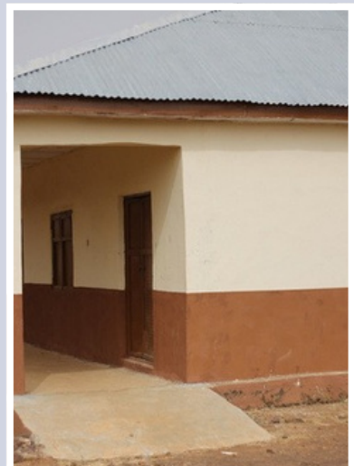
Newly renovated block of classroom by the AGILE Project at Government Day Secondary School (GDSS) Dalijan, Gwandu Local Government Area, Kebbi State
