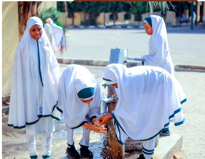
Learners at Girls Science and Technical College, Mairo Tijjani, in Kano using AGILE provided water facility.
