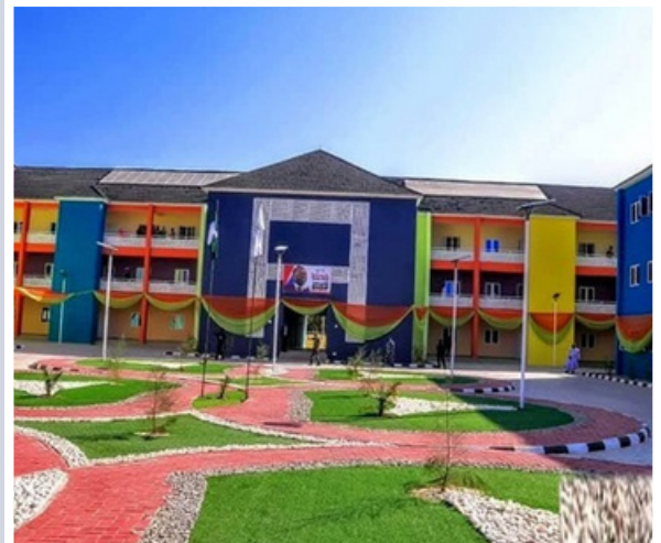
Kolugumna Secondary Secondary School in Borno State reconstructed by the AGILE Project after it was devastated by 10th September 2024 flood
