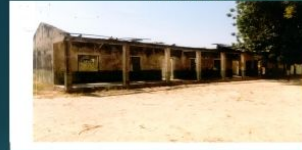
JSS Bahindi Before Renovation
