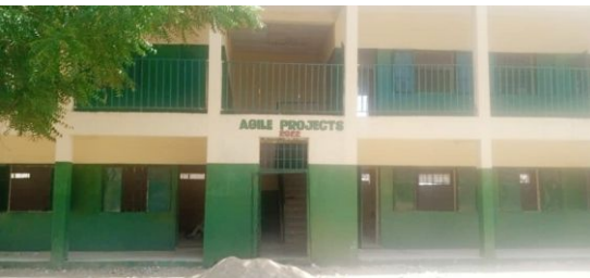
Renovated Government Secondary school, Sheka
