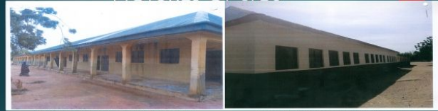
GDSS Mudi Kamba Before Renovation
