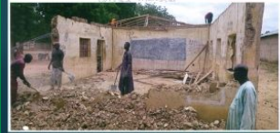
GDSS Mungadi Before Renovation
