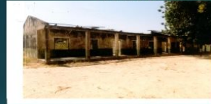
JSS Bahindi Before Renovation
