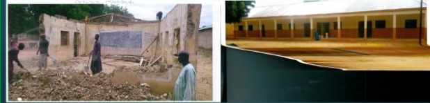
GDSS Mungadi Before Renovation
