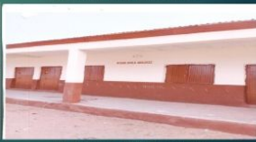
JSS Bandam After Renovation
