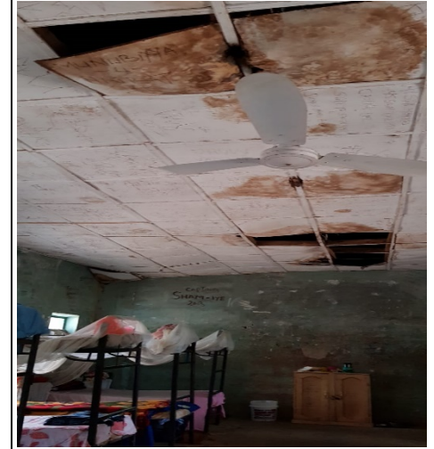
Plates 15: Rotting and Falling ceiling in a girl's hostel, walls and floors cracked and very old
