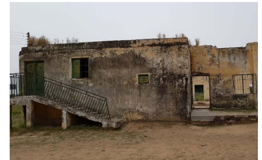
Plates 12: Abandoned building in a school
